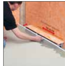
=> 4. Ajuster le support de caniveau
